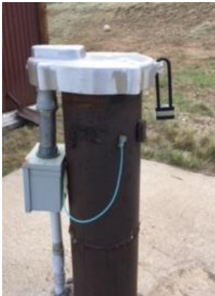
Image 1: Security padlock installed on Well 2 wellhead
